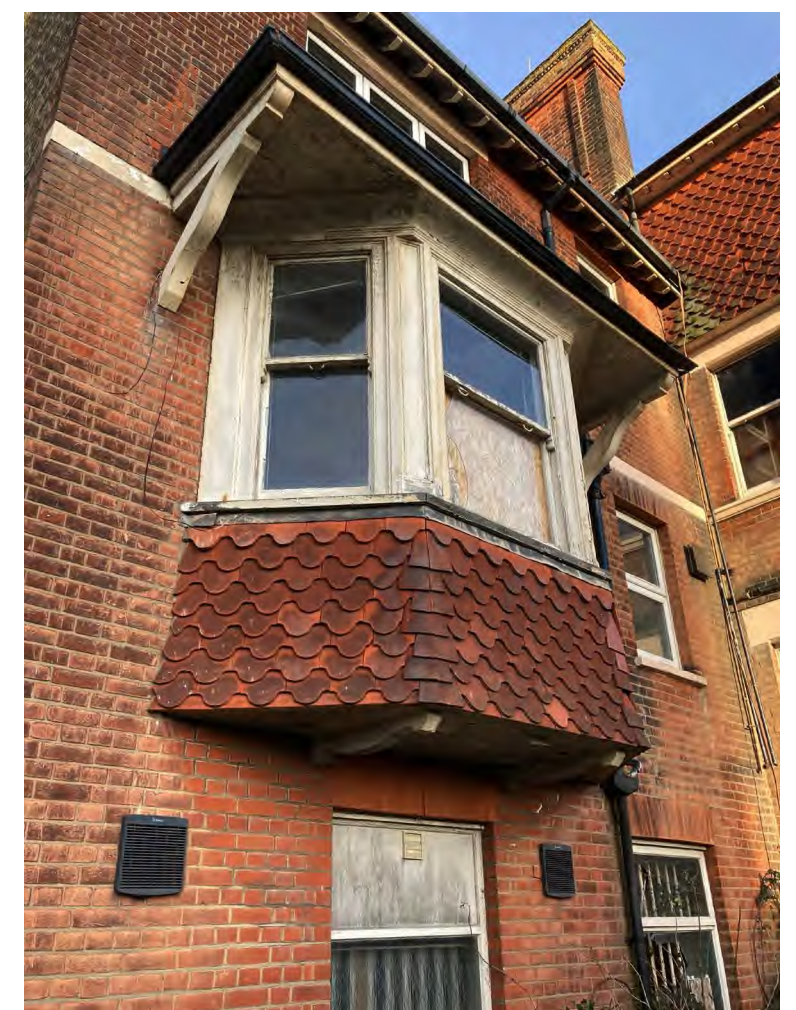
Site photograph detailing existing timber frame sash windows
