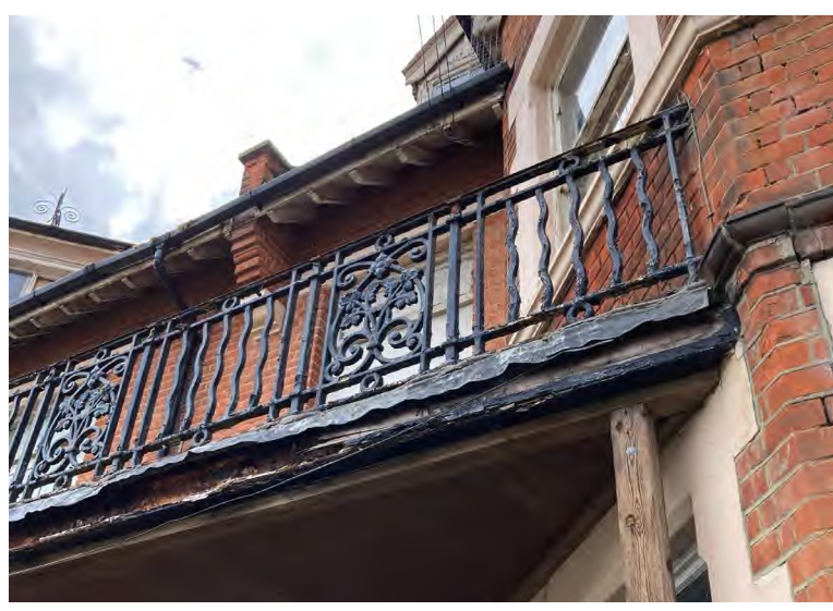
Site photograph detailing existing feature balustrade on site
